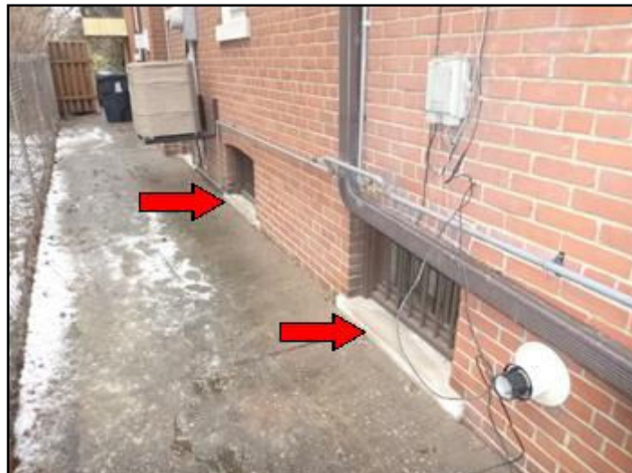
windows at grade level (north side)
