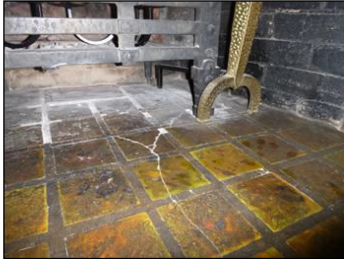
Firebox gaps/cracks
