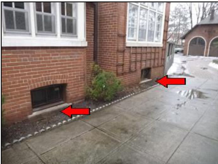
windows at grade level (south side)
