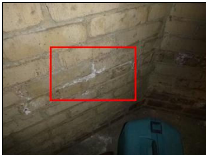
Efflorescence
